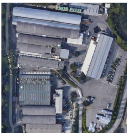
Figure 1: Tenax S.p.A production plant – Viganò (LC)
